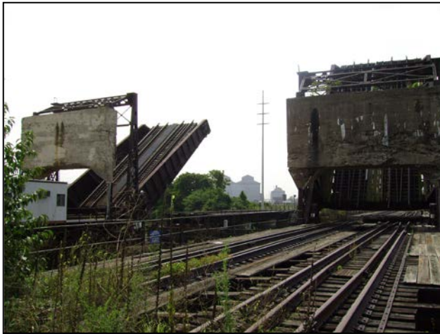
(The B&O Railroad bridge over Darby Creek, between Ridley and Tinicum. This is an example of an overhead-counterweight bascule bridge likely designed by Joseph Strauss in 1916).
